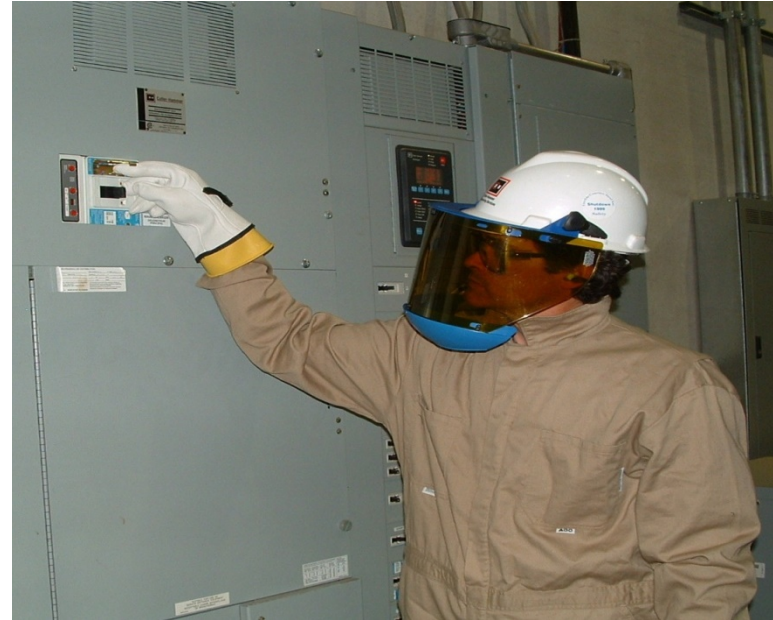
Good - All of Body Protected Toward the Arc Flash Area
