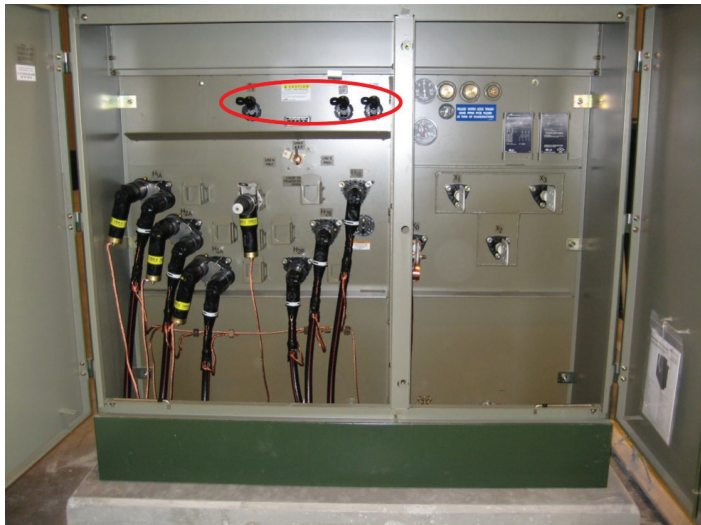
Figure 2 – Example of pad-mount transformer with primary bayonet style fusing.
