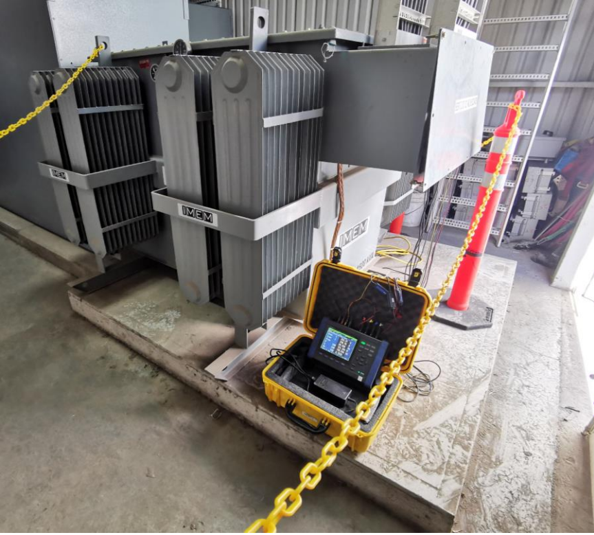
Power Quality study with portable analyzer
